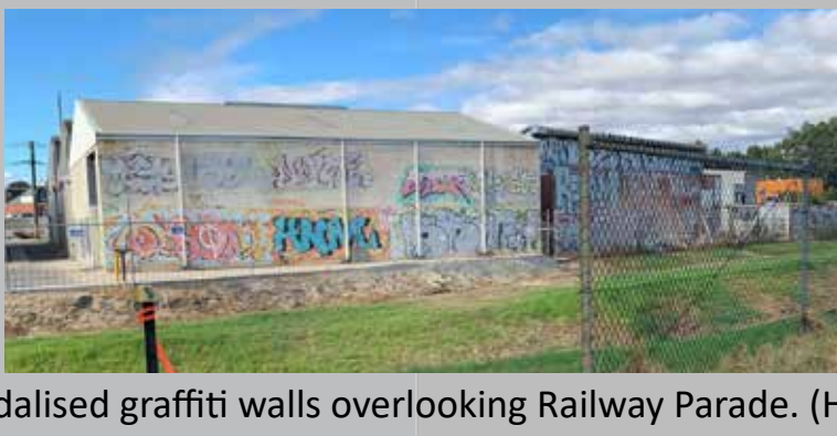
Vandalised graffiti walls overlooking Railway Parade. (Hunt 2019)
